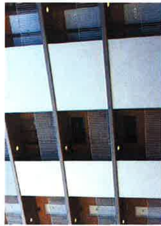
Example of LC1 in-fill between CR1 off form concrete slab
