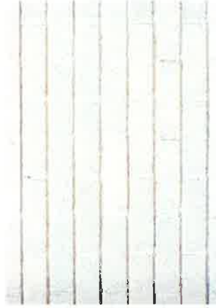
BWK - light coloured brickwork
