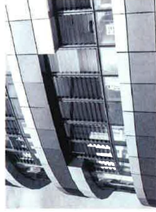
W - Aluminium framed windows - light grey finish (example)
