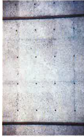
CR1 - Class 2 off-form concrete
